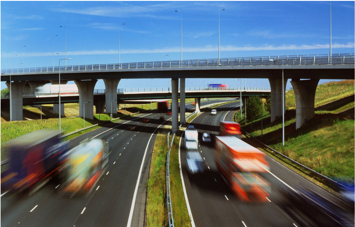
Photo: Road Management Services (Darrington) Limited
